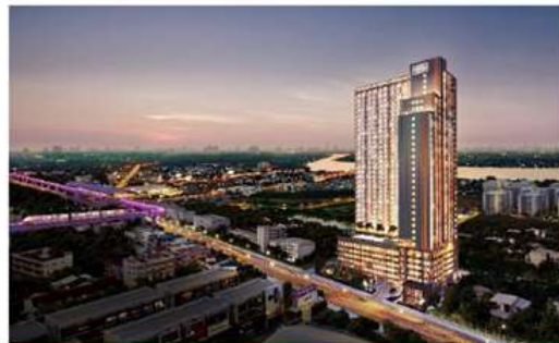
2. Niche ID @ Pakkret Station
